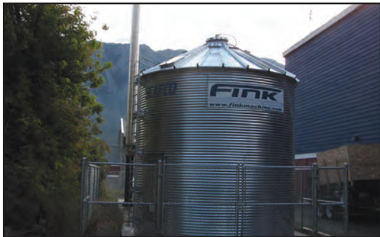
Figure 7 - Pellet Storage Silo
