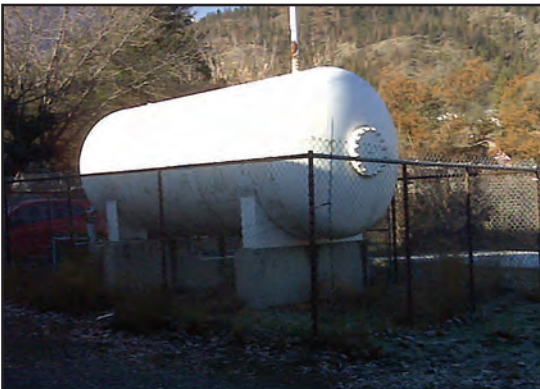
Figure 4 - Old Propane Storage Tank
