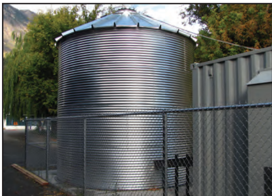
Figure 14 - Auger from Pellet Silo into Boiler Container
